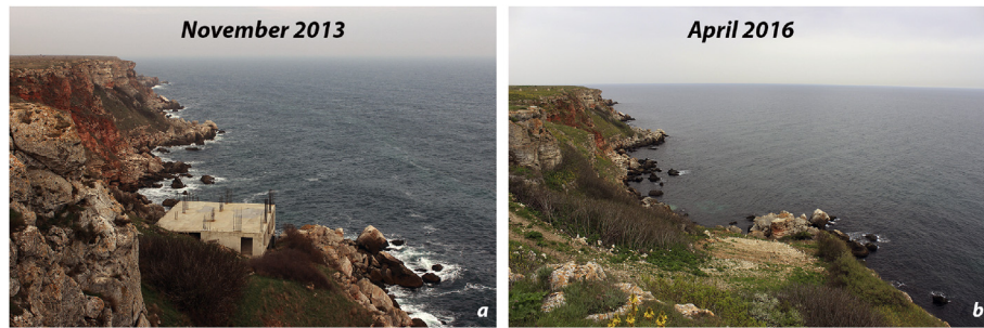
Fig. 9. a) Construction in Yaylata Protected Site and Archaeological Reserve in 2013; b) Removed construction in 2016.
